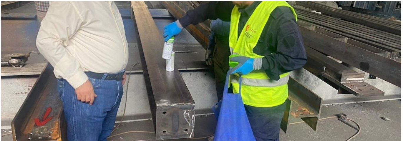
Hands-on oversight: inspection at the fabrication shop
