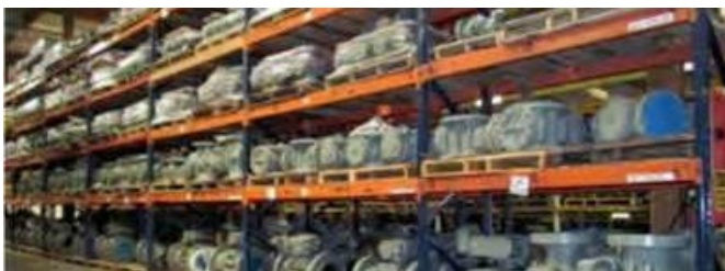
Pipeline valves, fittings and spares
