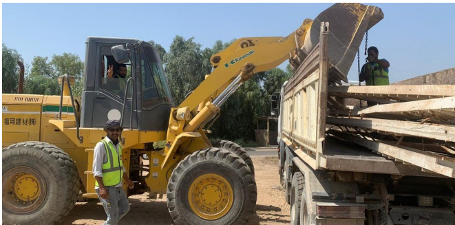
Site clearance and material loading
