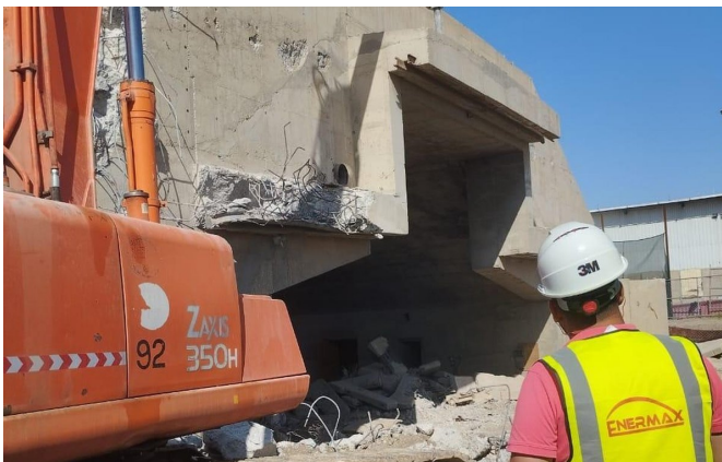
Demolition of a hardened aircraft shelter (HAS-1), Baghdad
